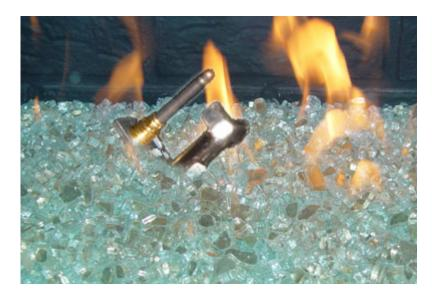
Now pour the Glassel over the top of everything, keeping the Thermocouple Assembly positioned just above the glass and directly over the rear burner pipe, as illustrated.
